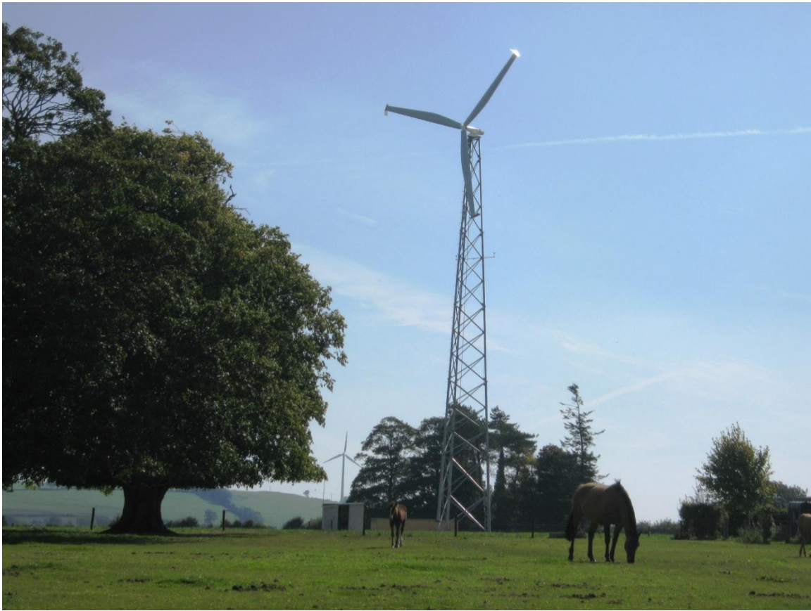
Figure 1: AOC 15/50 on lattice tower (Gurteen College, Ireland).
